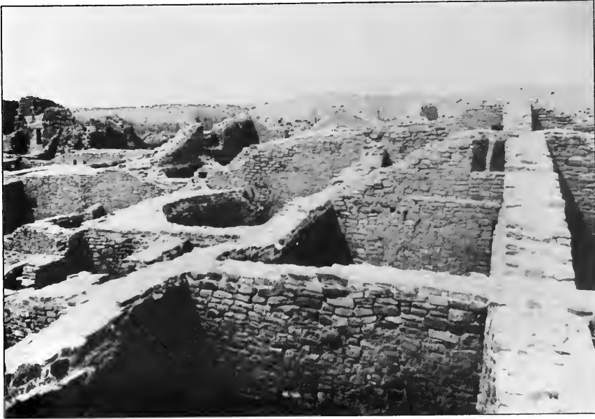
Figure 12.1. View over northeast corner of West Ruin showing cement wall capping.
